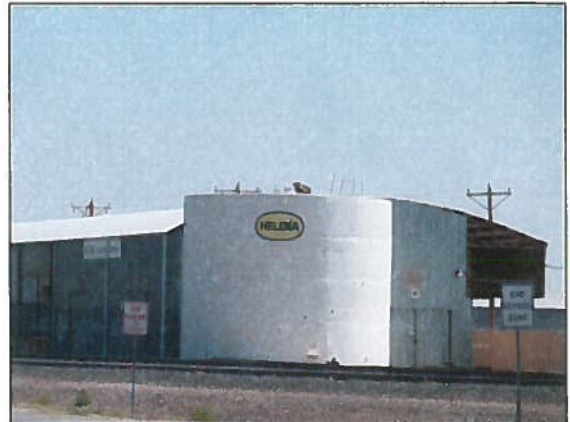
One of the many chemical storage units on site at the Helena Chemical facility in Mesquite.
